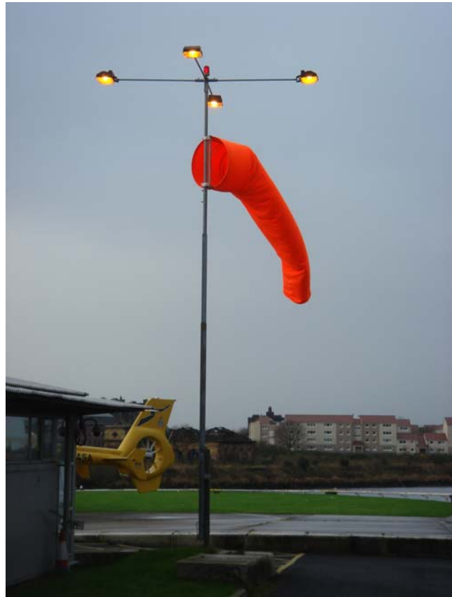
Glasgow SECC Heliport
